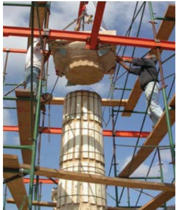
Figure 16: A column (of new material) at the SE corner of the peristasis of the temple of "Athena" crowned by its Doric capital.
