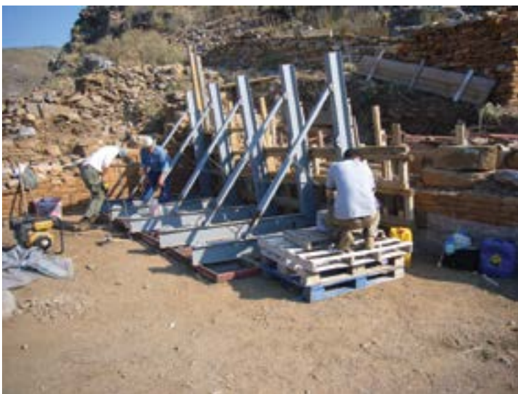
Figure 19: Pushing back the wall of building D into its original, vertical position.
