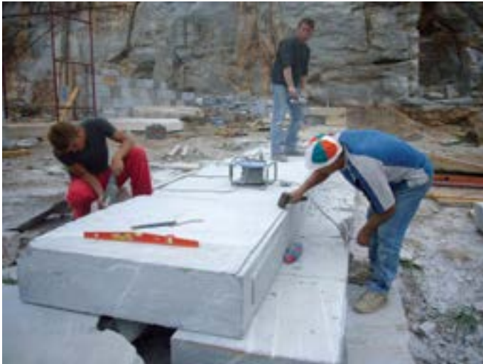
Figure 8: Temple of Apollo. Restoration of the krepis and of the steps to the pronaos.
